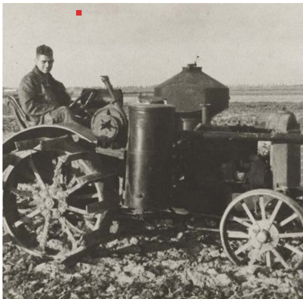
MacCormic tractor met houtgasgenerator
